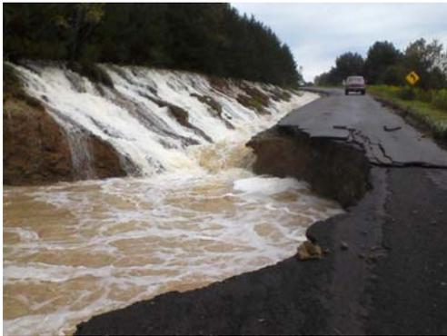
Photos of Bailey Hollow Road Flood Damage (2011, Town of Maine)
