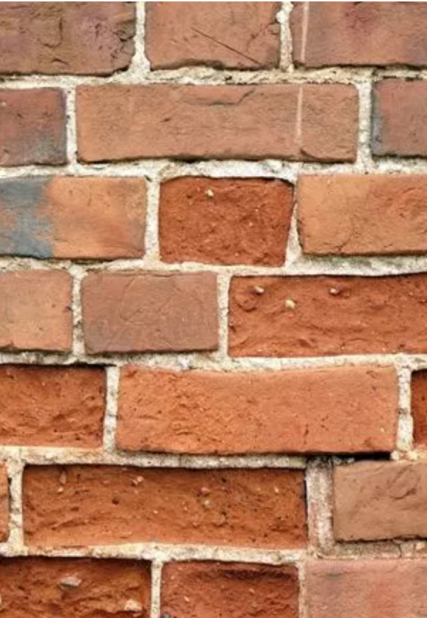
EVIDENCE OF BRICK SPALLING.
