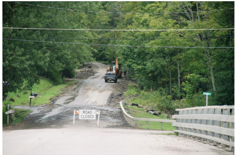
2011 Flood Damage to Road
