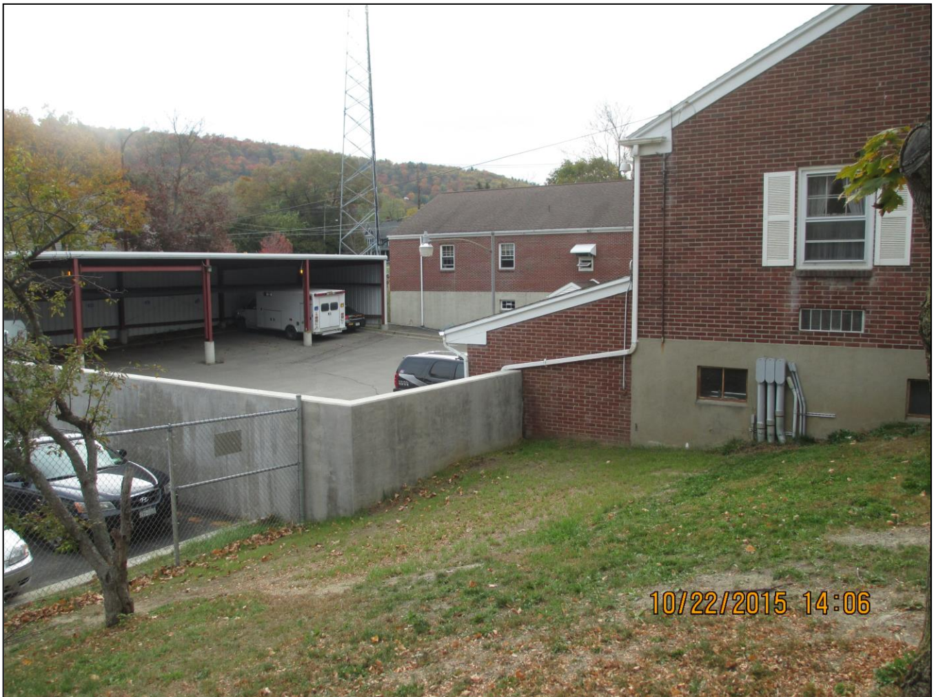
7-foot Floodwall built to protect the Town Hall from future flooding
