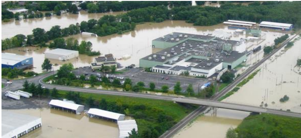
Flooding near Colesville Road Extension and Spud Lane (September, 2011)
