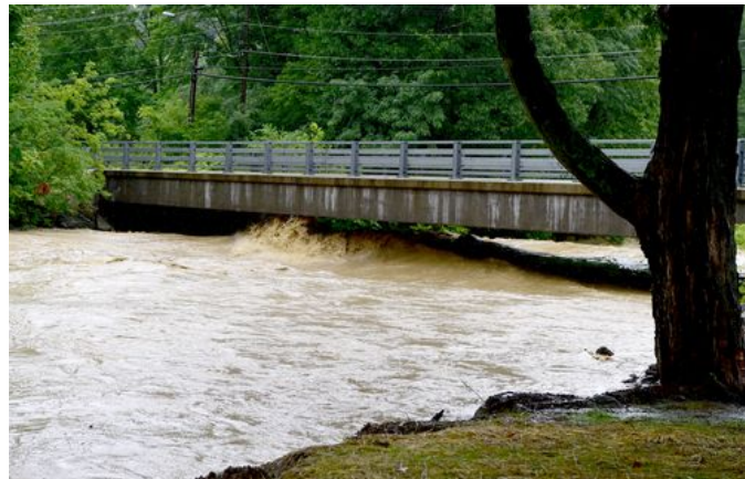
Concerns over Choconut Creek flooding prompted officials to close roads and advise evacuation for certain areas of Vestal on August 14, 2018 Source: Pressconnects 2019
