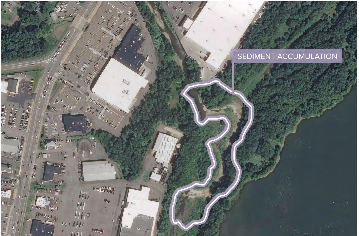
Existing Site Conditions Photo Credits: EagleView
