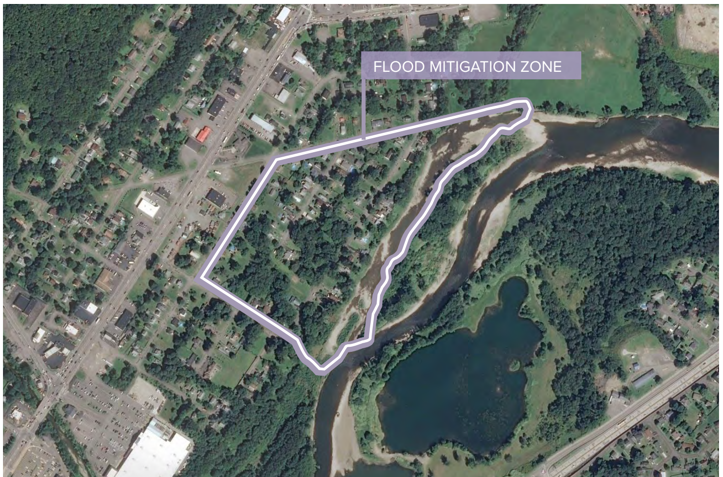
Existing Site Conditions Photo Credits: EagleView
