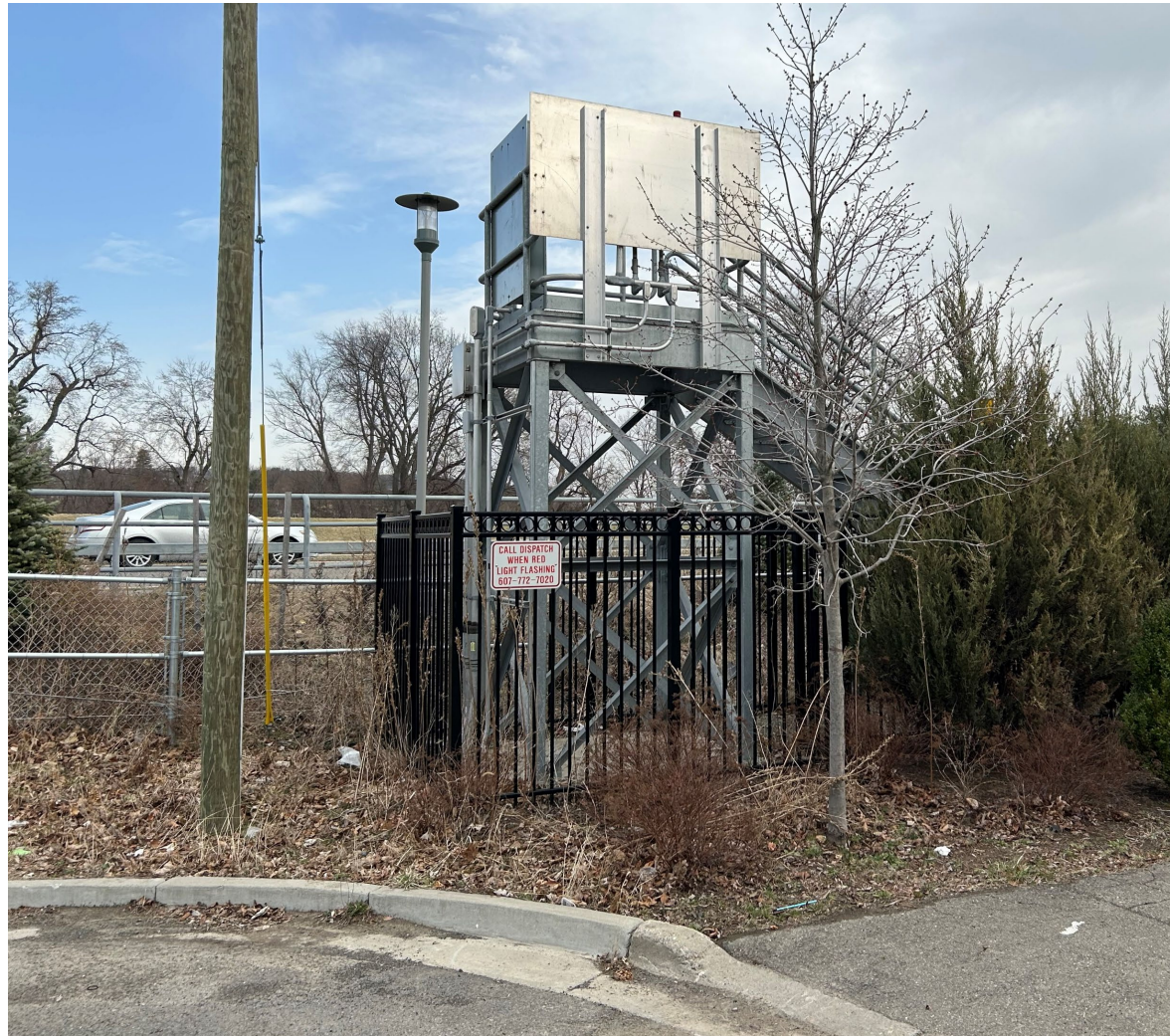
Sewer pump station elevated controls for two 5 horsepower pumps
