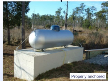
Anchored Propane Tank
