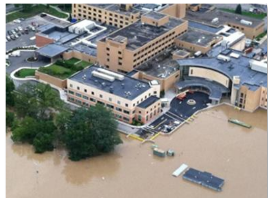
A floodwall protected Our Lady of Lourdes Hospital in Binghamton, New York during Tropical Storm Lee in 2011 Photo by FEMA.
