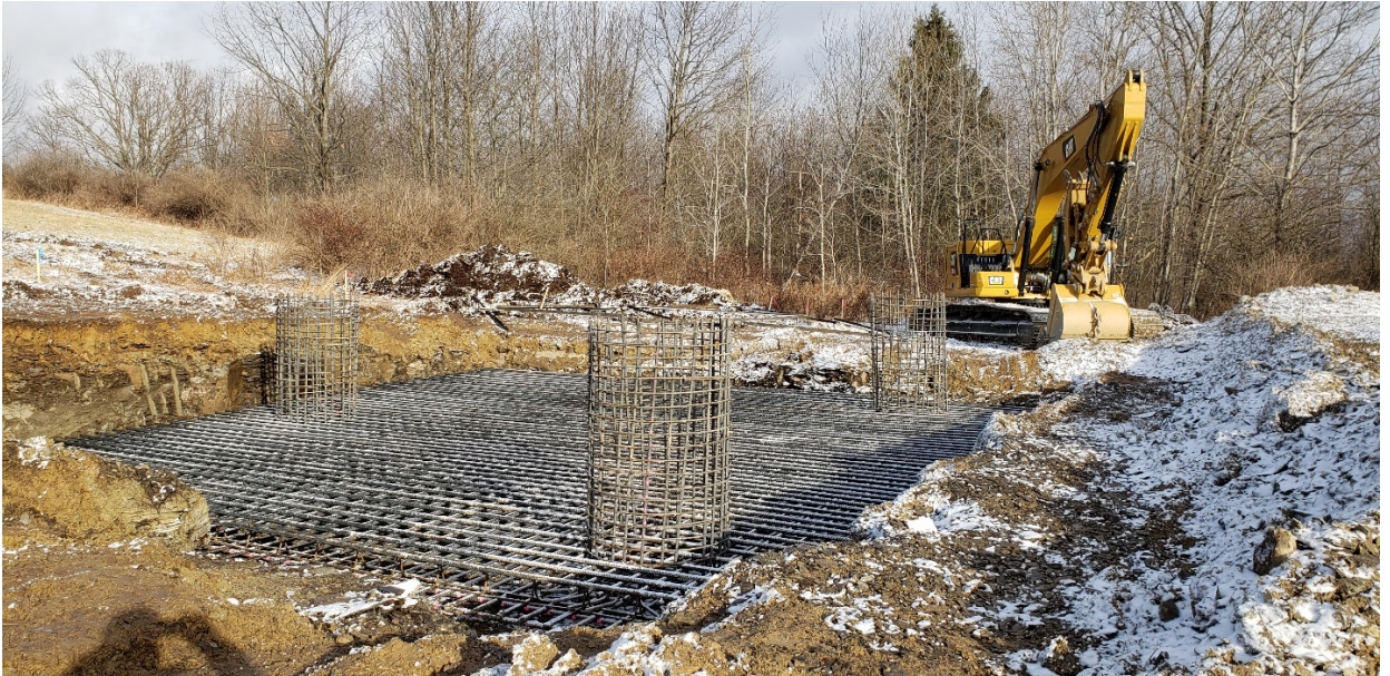
Nabinger Hill – Rebar for tower foundation.
