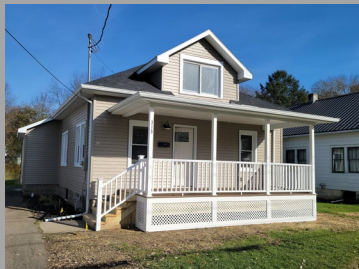
313 Marion Street, Town of Vestal
