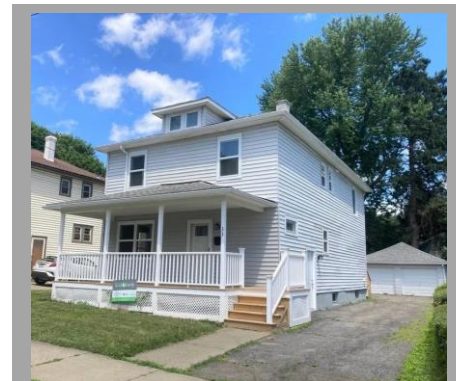
33 Linden Street, City of Binghamton
