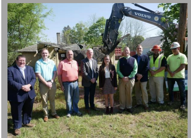
2300 Owego Rd., Town of Vestal pre-demolition press conference with County, Town and Land Bank Officials
