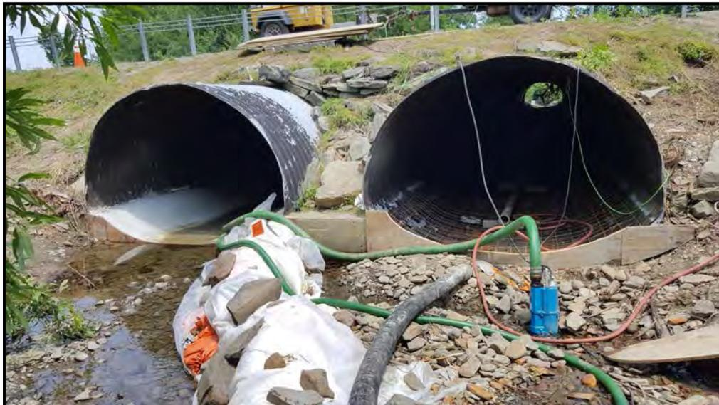
***Photo #2:*** BIN 3371100 Broome Corporate Drive Bridge – placement of concrete inverts – Summer 2018.
