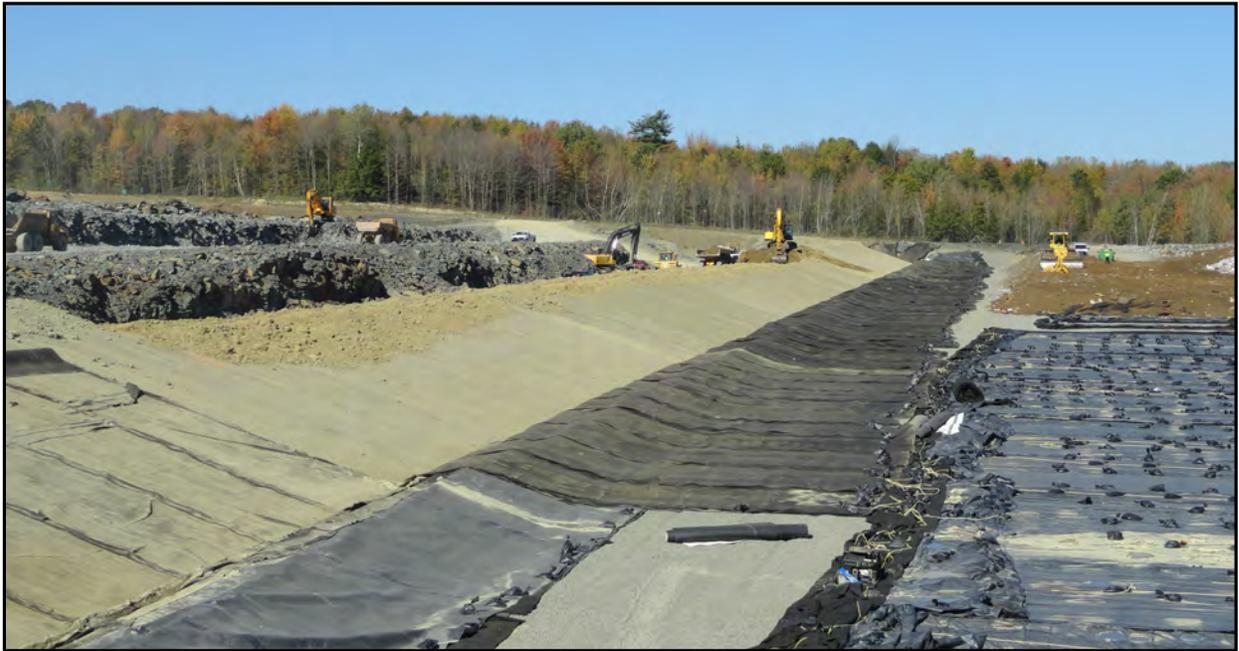
Photo 7: Cell 3-4 Berm Reconstruction
