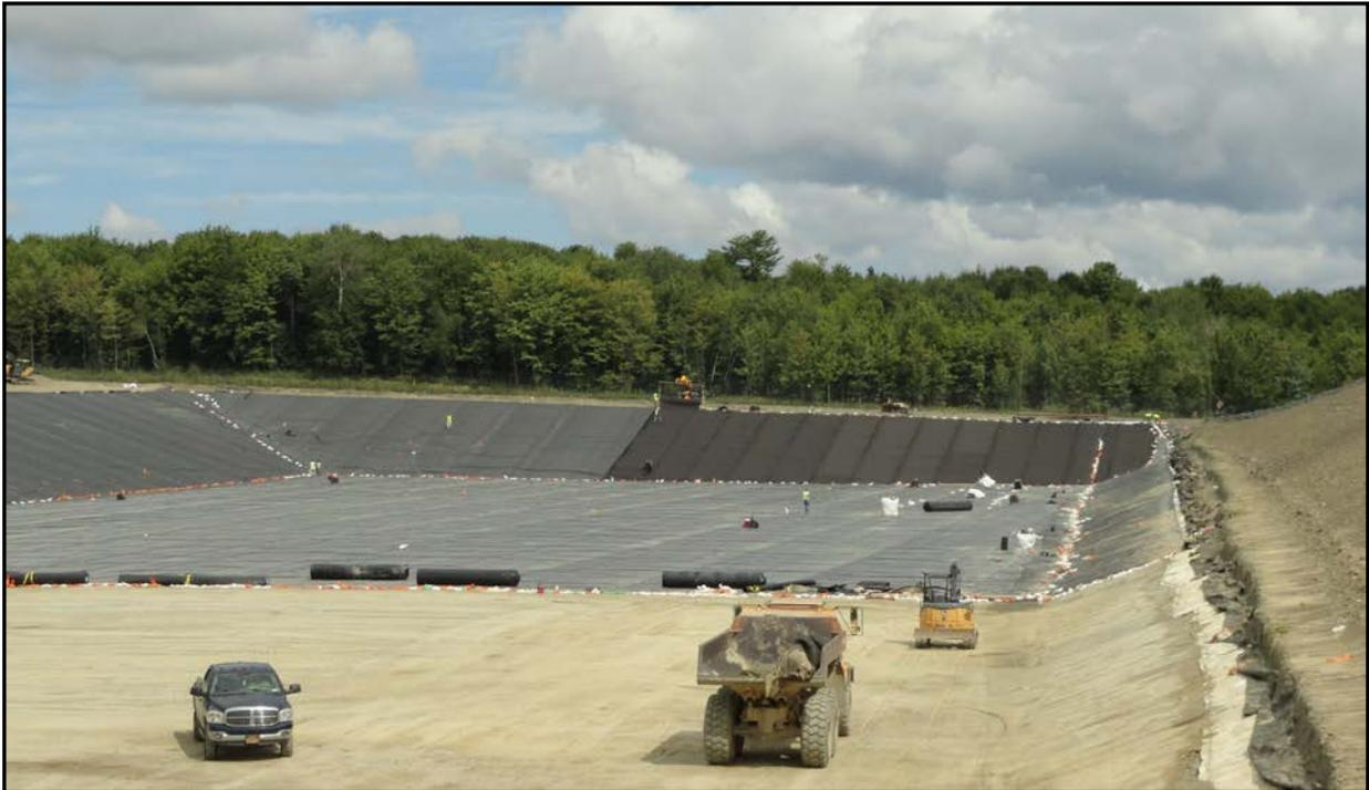
Photo 7: Section IV -Cell 4 Liner Construction
