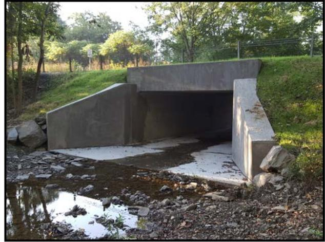
**Photos #4 & #5:** CIN 40-2.01 Colesville Road Culvert – Class D concrete wingwall & headwall repairs (before and after repairs) – typical of several large culvert repairs completed in 2019.
