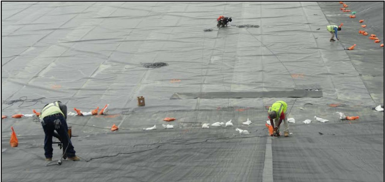
Photo 6: Landfill Section IV- Cell 4 Welding of Liner Seams
