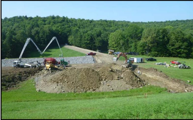
***Photos #6, #7, & #8:*** Construction of Watershed Site 9A improvements and upgrades – placement of a concrete cutoff wall, raising of the dam crest, and armoring spillway embankments - Summer 2019,
