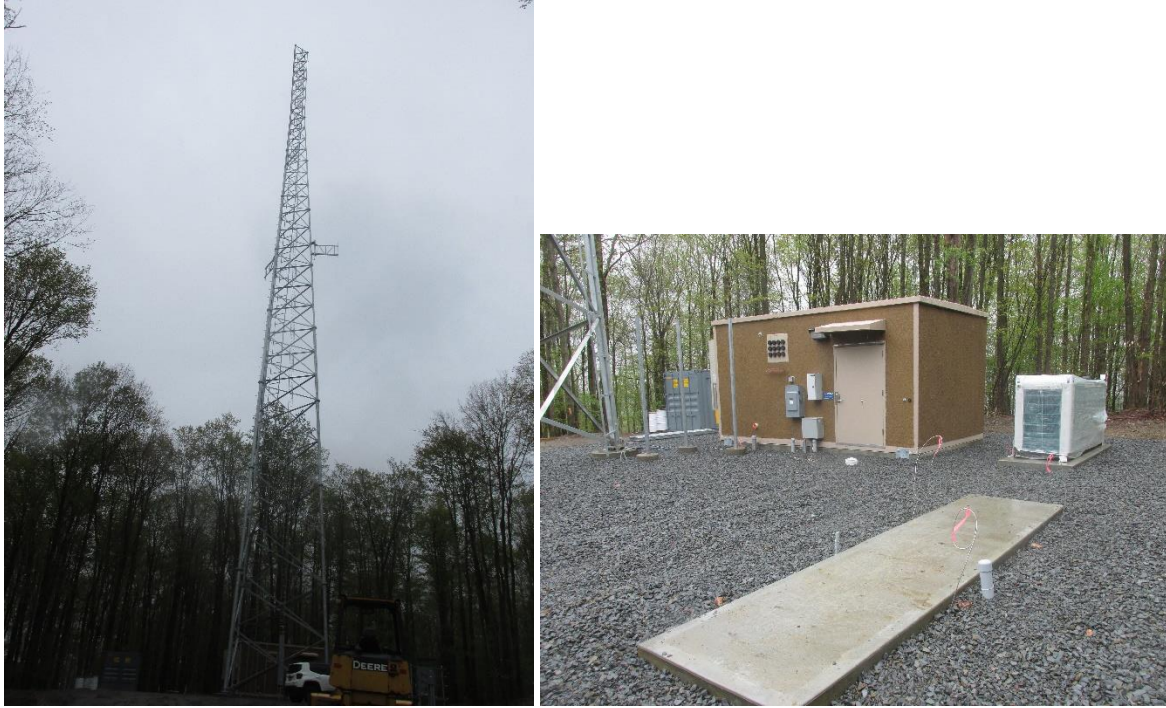
Maine Tower Site and Compound
