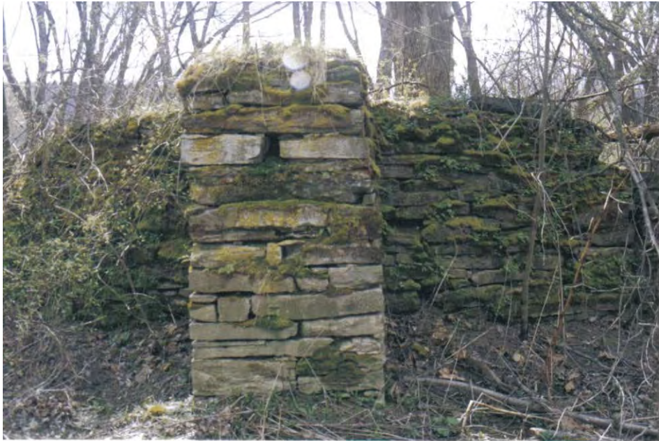
Details of the east abutment
