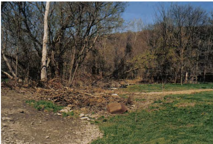
19 Old State Road - looking northeast from the backyard the, towpath is on the left. Debris fills the remains of the prism.
