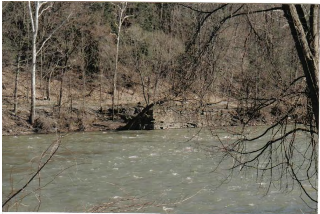
The guard lock seen from the west bank of the Chenango River.
