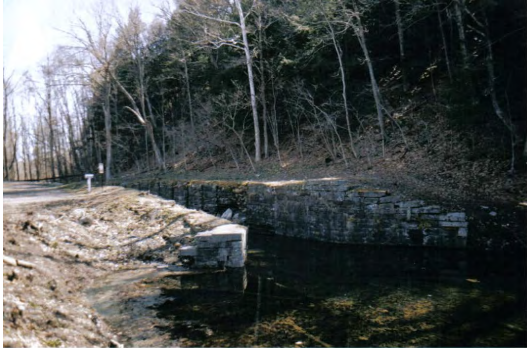
Water from the Chenango River entered the canal here, just south of Lock 107.
