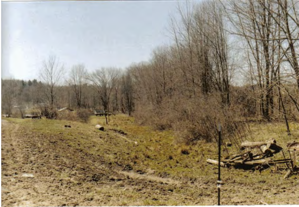
Behind the barn the canal prism has been dammed and the prism is dry to the south
