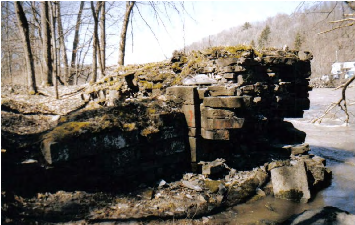
Above - looking south down the water filled prism from the west wing wall of Lock 107. Below - remains of the guard lock which allowed water from the river to feed the canal .
