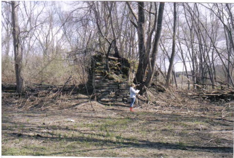
Looking west - the remains of the east abutment.
