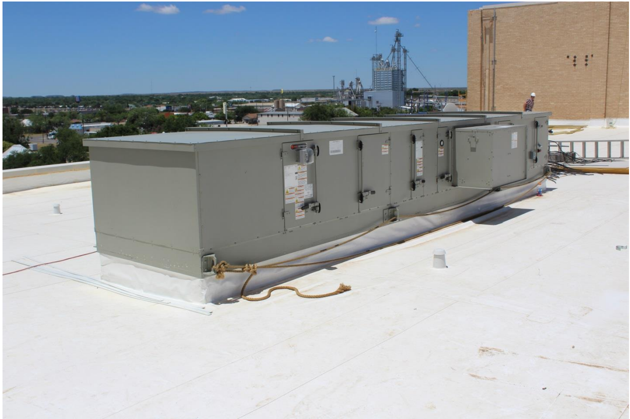
Example of Low Noise Fan Coil on Roof of a Theatre
