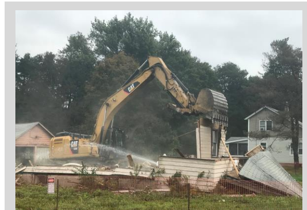
2977 NYS Route 26, Town of Maine
